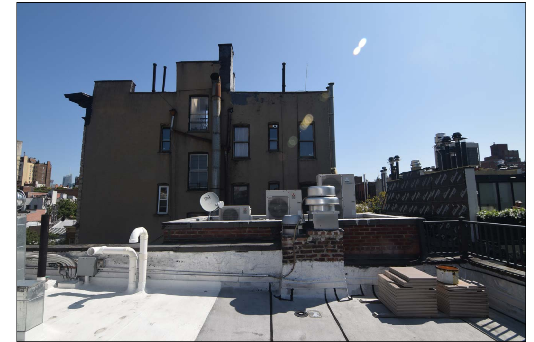
3 52 BANK - 6 STOREY BUILDING TO THE EAST
