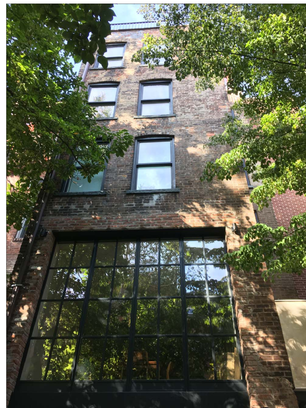
5 SUBJECT PREMISES - REAR WALL
