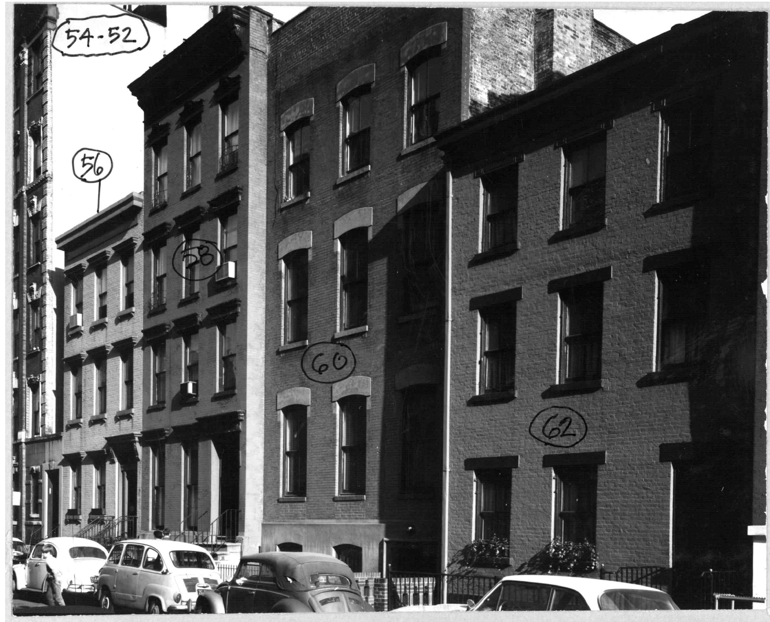
2 1969 HISTORICAL DESIGNATION LPC PHOTOGRAPH - LOOKING SOUTHEAST
