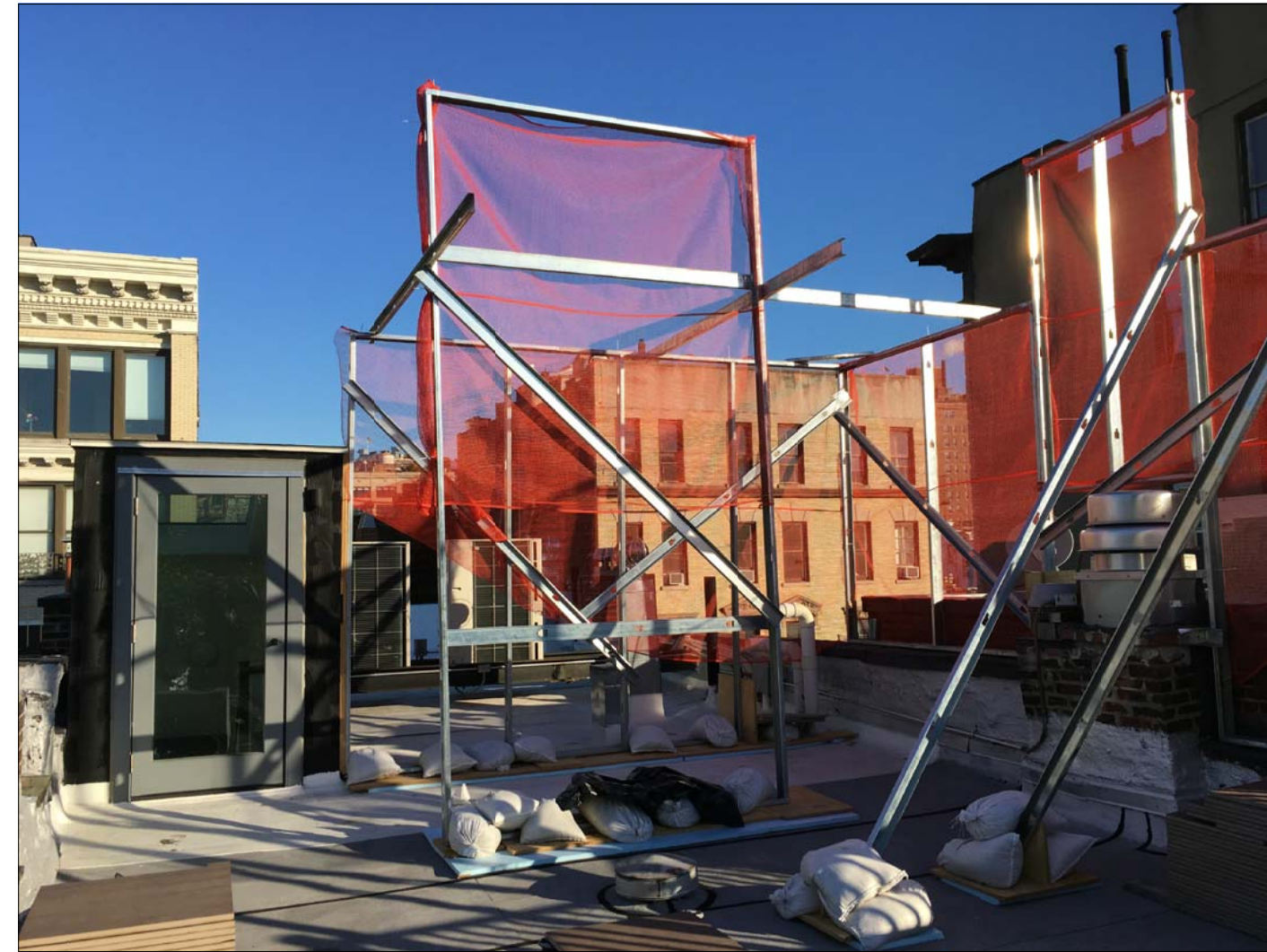
3 VIEW NORTHEAST @ ROOF
