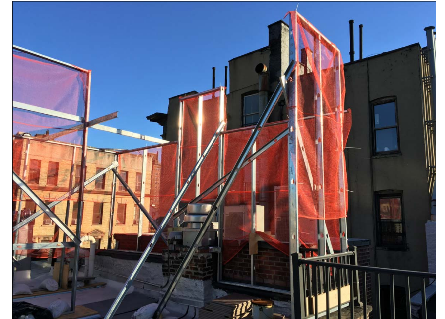
4 VIEW EAST @ ROOF
