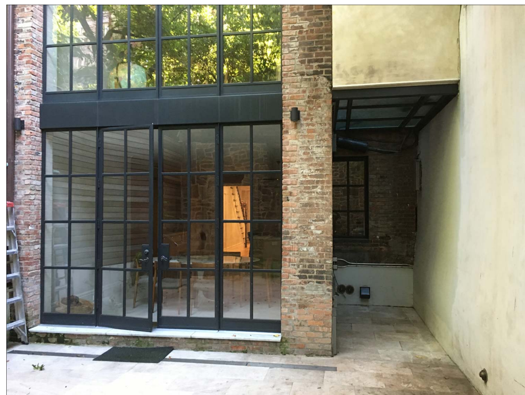
4 SUBJECT PREMISES @ CELLAR
