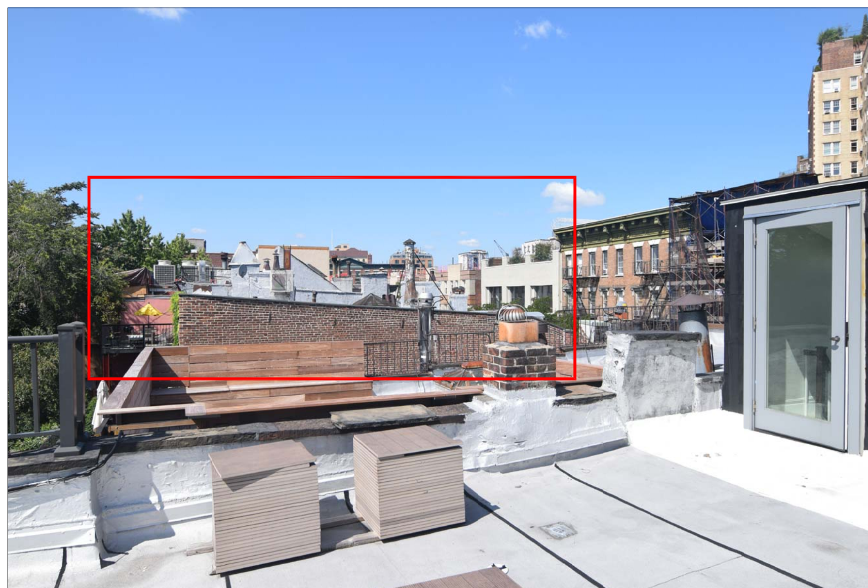
6 70 BANK - 4 STORY w/ROOFTOP ADDITION
